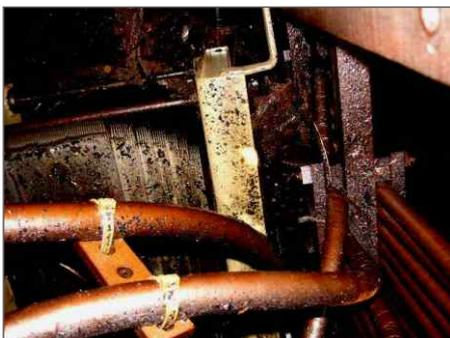
Short circuit due to high moisture content of the insulating oil
